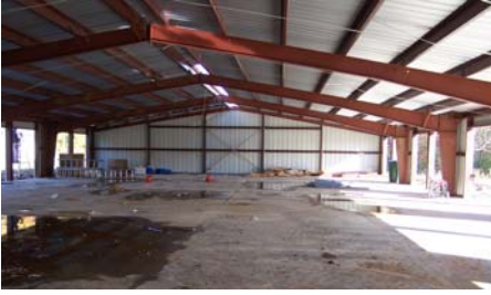
Interior construction photo showing steel frame before interior partitions installed.
