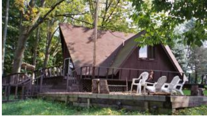
Side view or West side of A-Frame.
