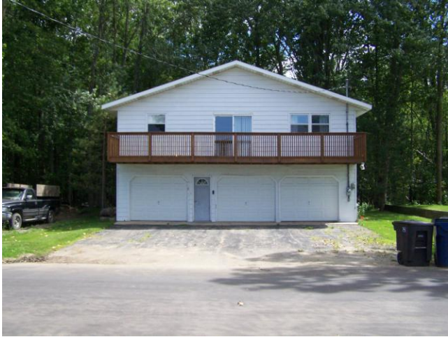
Detached garage on back lot with apartment above.
