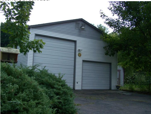
Backside lot area 24 x31' pole barn.
