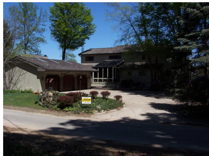
View from the roadside.
