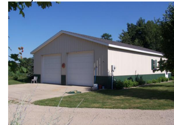
30 x 48', work bench, wood burner.
