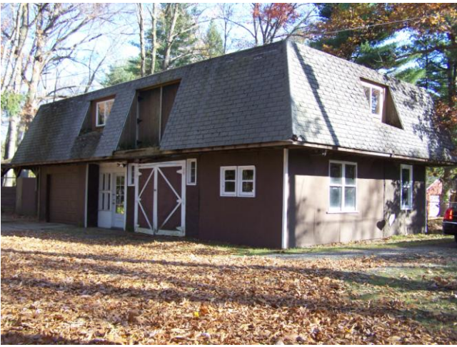
2 1/2 Car Detached Garage & overhead Loft
